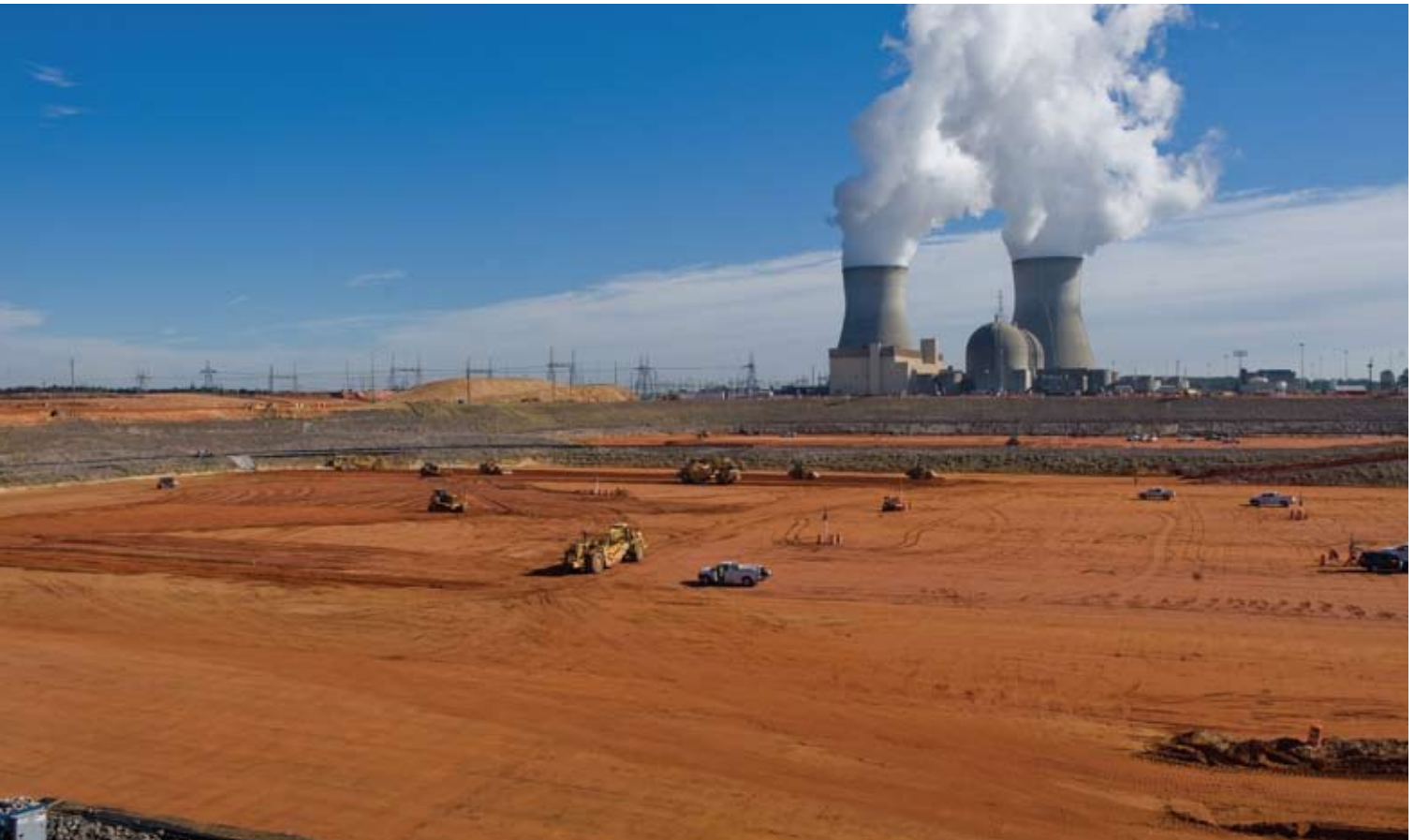
Two nuclear units are being added to Plant Vogtle in eastern Georgia.
