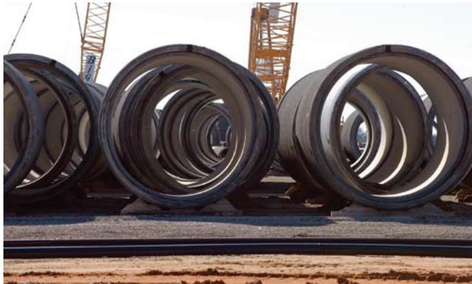
Unassembled circulating-water piping for the two new units.
