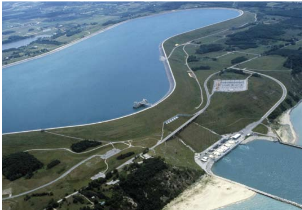
The Ludington plant's 27-billion-gallon reservoir.
