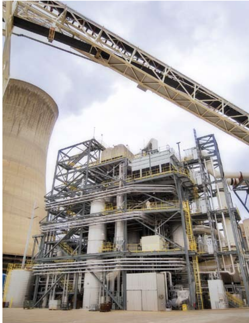
The CCS project captures up to 90 percent of the CO 2 from a 20-MW portion of the plant's flue gas.
