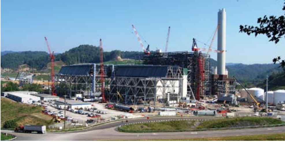
The Virginia Hybrid Energy Center, currently under construction in Southwest Virginia, is designed to use biomass for up to 20 percent of its fuel supply.
